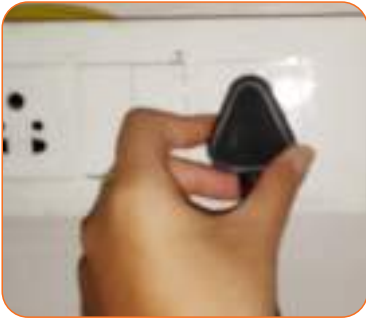
Figure 4.1.9 : Powering on the main supply
