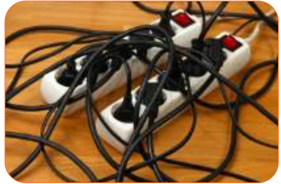
Figure 6.1.7 : Overloaded extension cords
