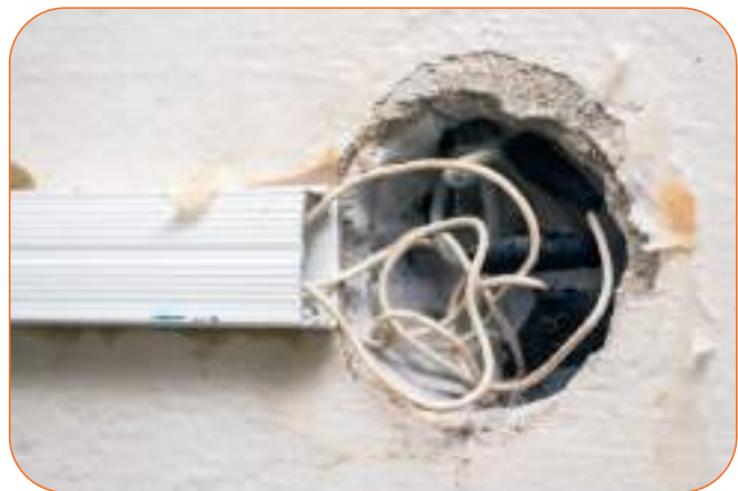
Figure 6.1.6: Be careful with exposed cables
